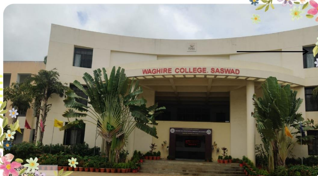
WAGHIRE COLLEGE OF ARTS, COMMERCE AND SCIENCE SASWAD, TAL-PURANDAR, PUNE 412301
