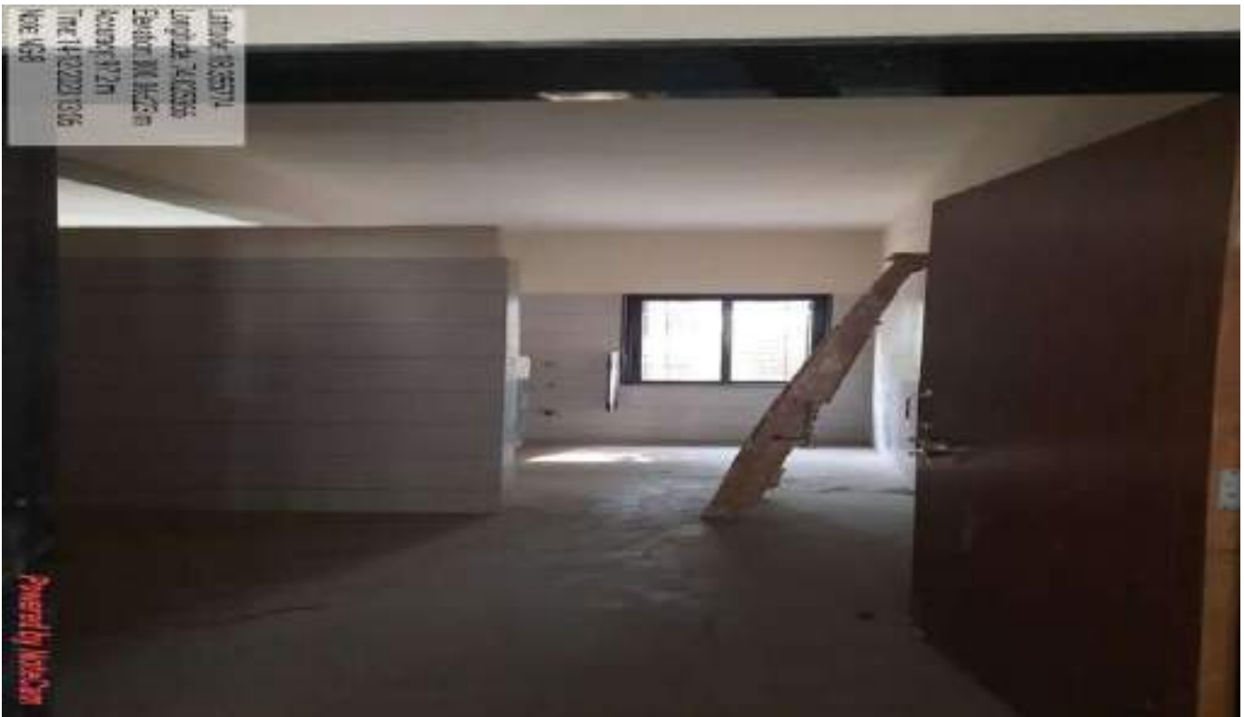
Figure 100 Common Wash Room NG-8
