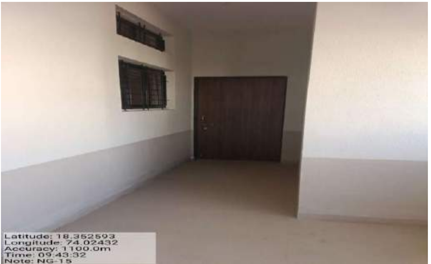
Figure 107 Common Wash Room NS 15
