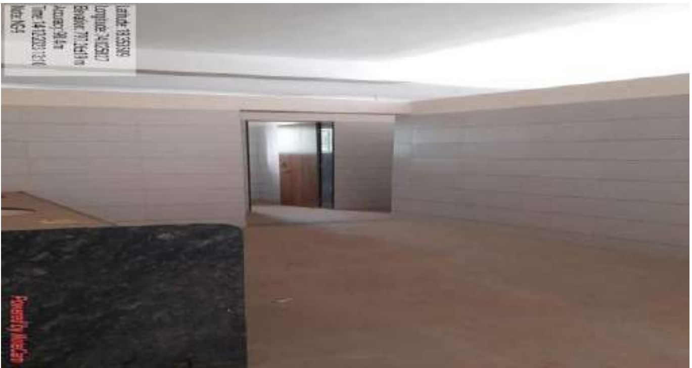
Figure 101 Common Wash Room NF-9
